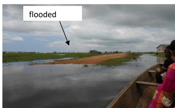
Photo 1 : Flooded roads to Kessounou
