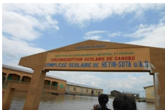
Photo 2. School Complex flooded Hetin-Sota
