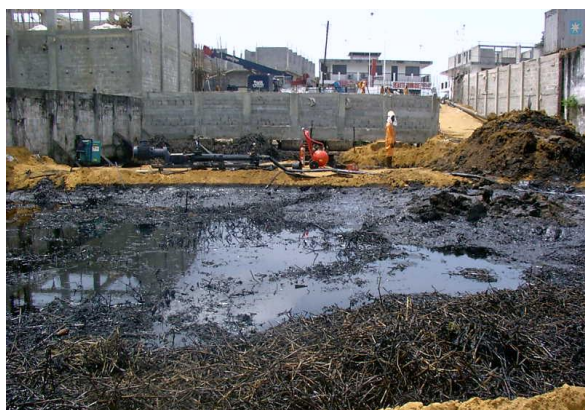
Photo 4 : zone principale de percement.
